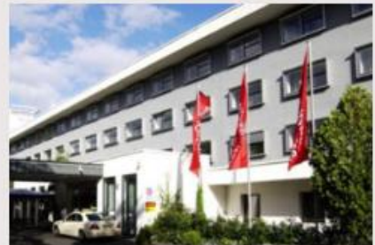
IntercityHotel Frankfurt Airport
